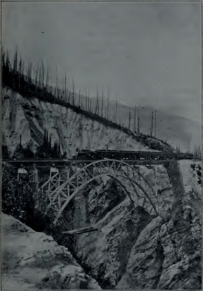
STONEY CREEK BRIDGE AND VANCOUVER-BOUND TRAIN.
